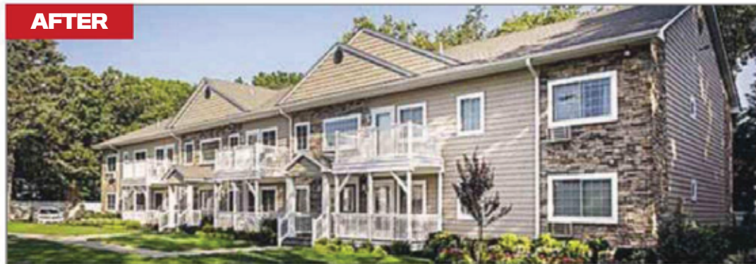
Part of Fairfield's work on the St. James development included renovating building exteriors.
