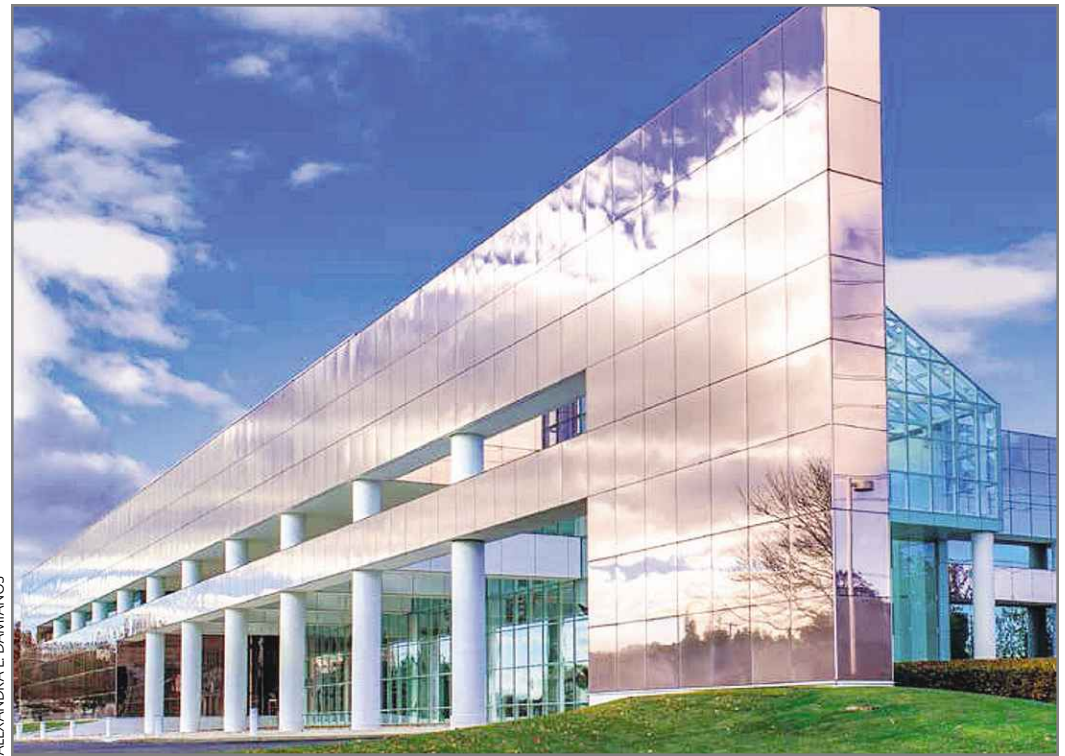
Damianos Realty Group of Smithtown reinvented this commercial building on Motor Parkway in Islandia.
