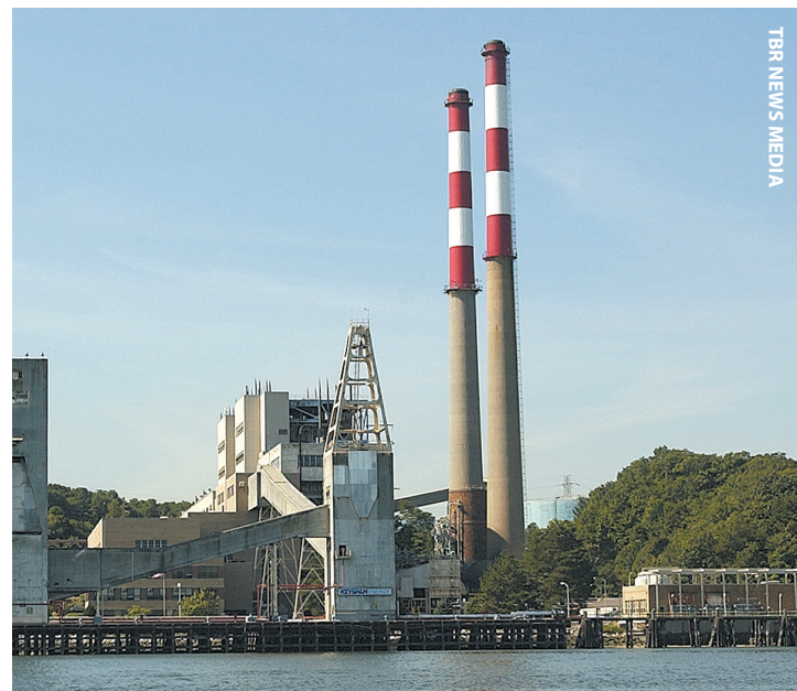
Port Jefferson's power plant located in the village.
