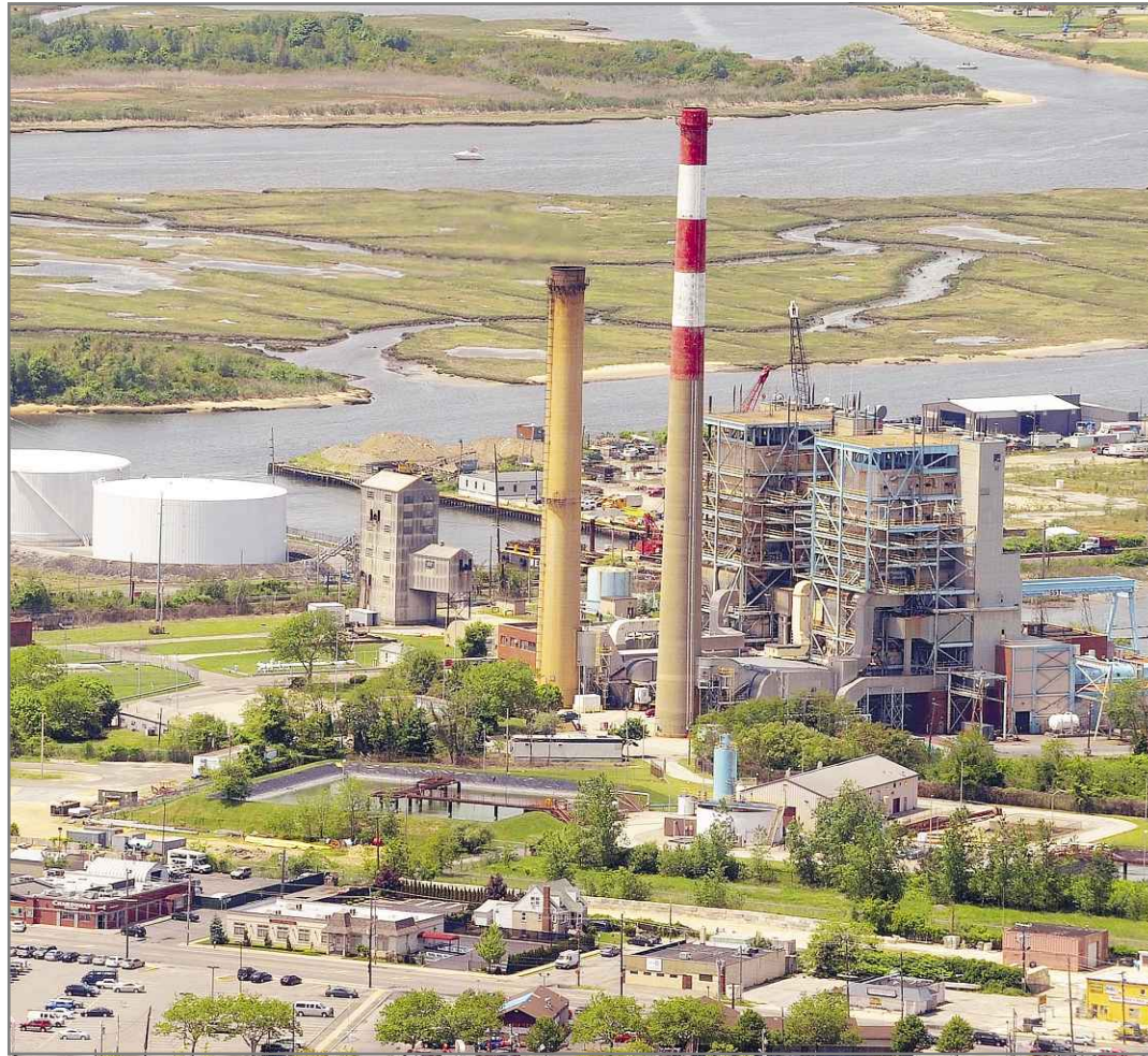
LIPA had challenged the property tax for the E.F. Barrett Power Plant in Island Park.
