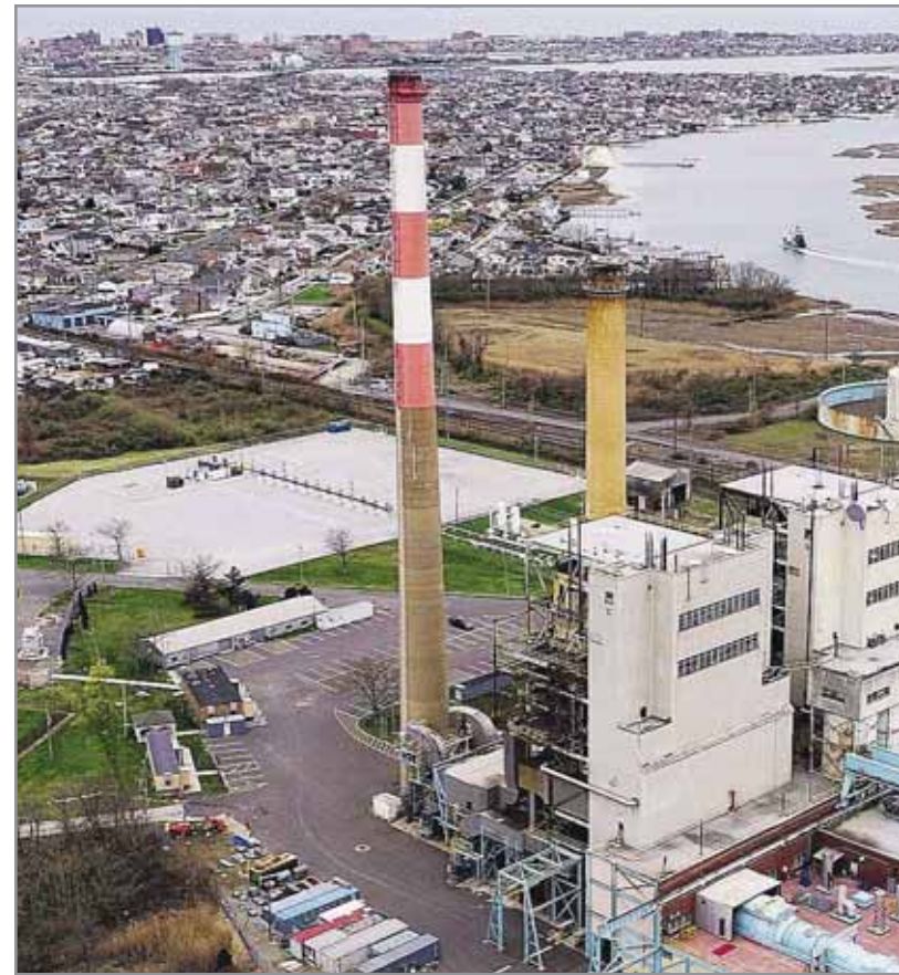
The E.F. Barrett Power Plant in Island Park is one of two LIPA plants
