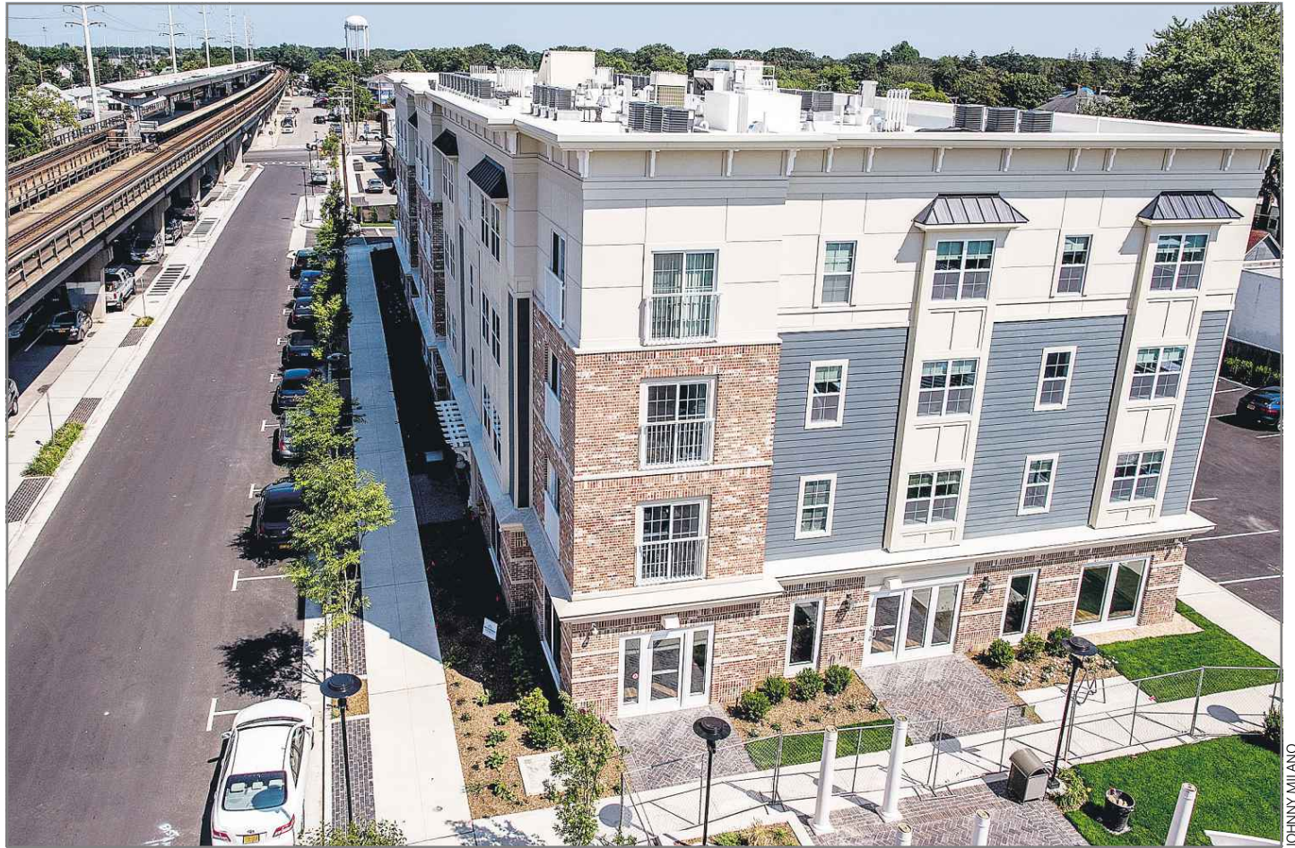
Conifer Realty's Copiague Commons, where builders are using materials designed to protect against flooding and major storms.
