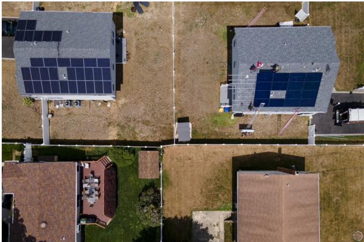
The Long Island hamlet of Massapequa, shown here, would be among the communities that would have to add new housing under a proposal by Gov. Kathy Hochul. | John Minchillo/AP Photo
